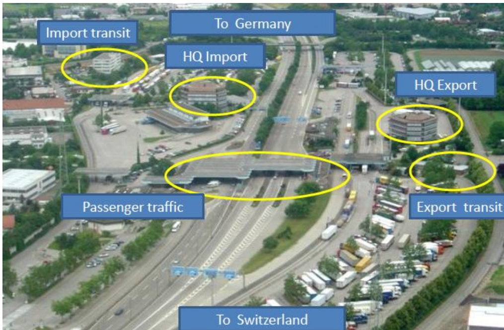
Figure 5: Common Juxtaposed border office at Basel / Weil am Rhein motorway
