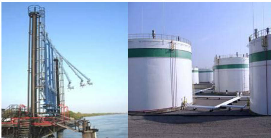
Figure 9: GIFP Oil Terminal Facilities
