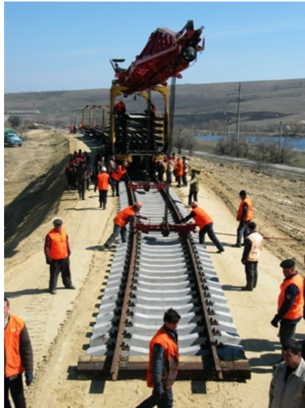
Figure 10: Construction of the Baku-Tbilisi-Kars Railway Line
