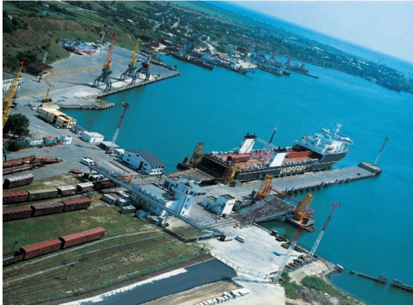
Figure 8: Ilyichevsk Railferry Terminal, Berths n°26, 27
