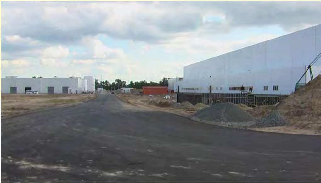
Figure 31: Boryspil Airport Commerce Park – Warehousing and Customs Terminal
