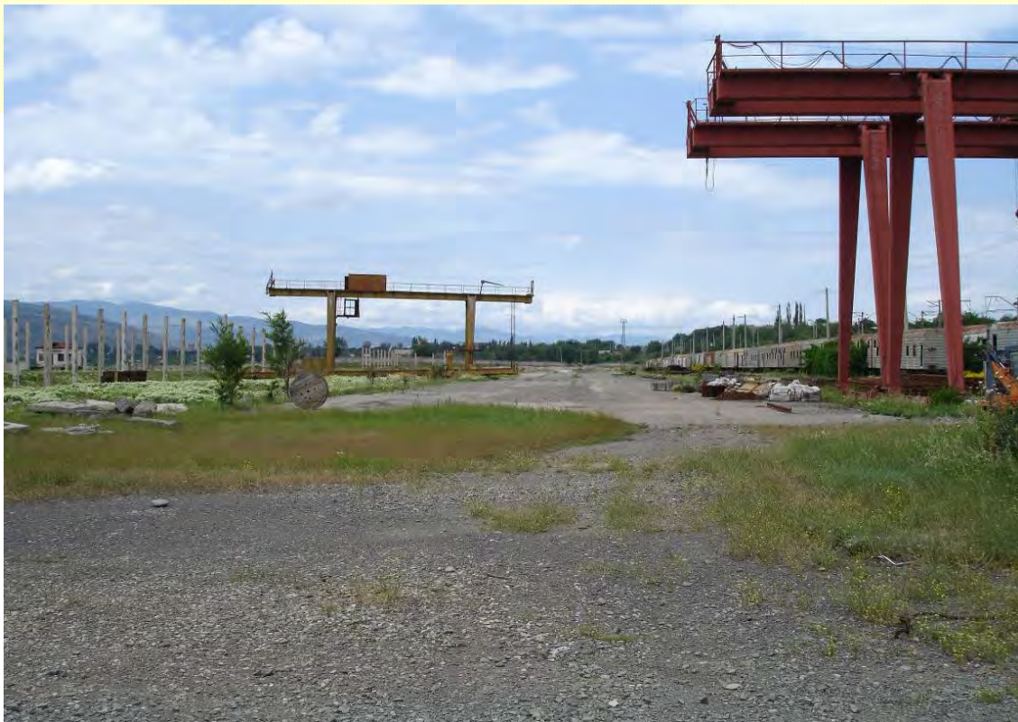
Figure 20: Railway Container Terminal – General View
