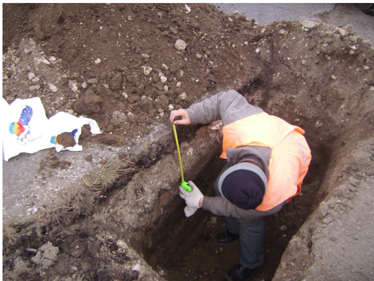
Figure 1-1. Trial pit excavation
