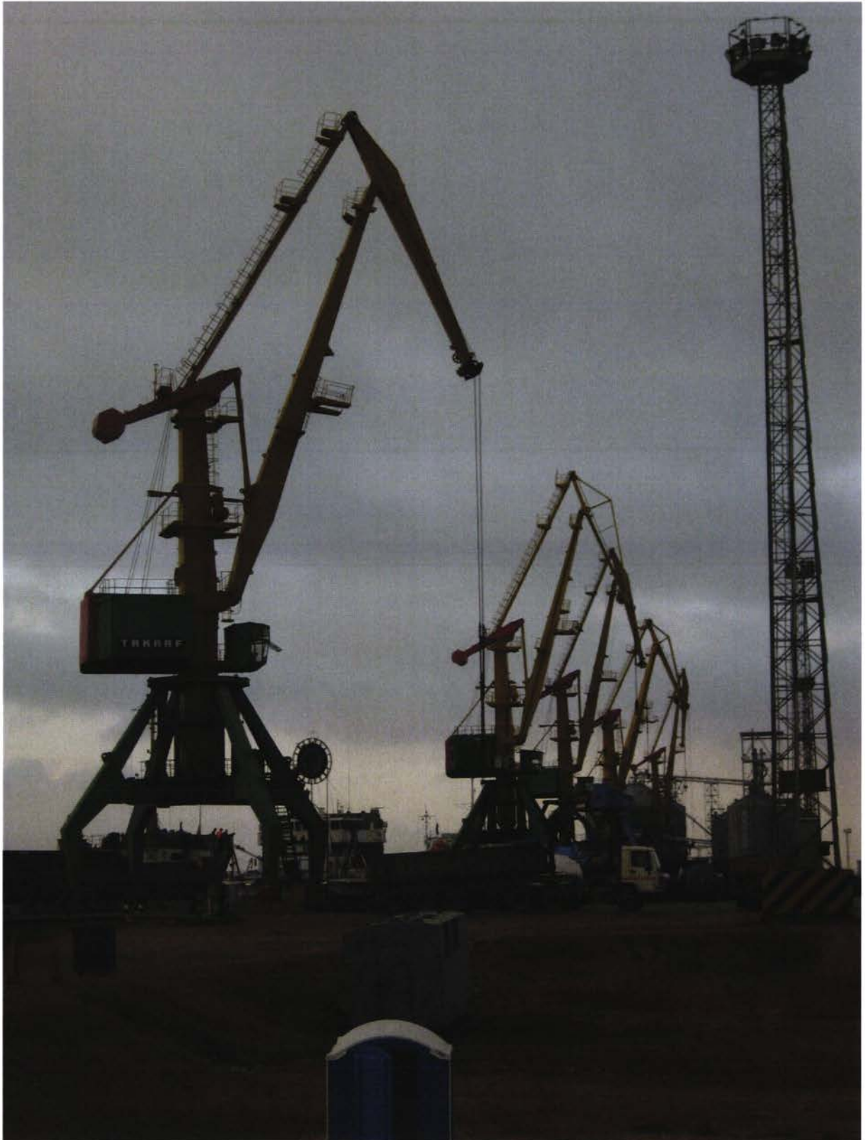
Cranes at berths 1-3
