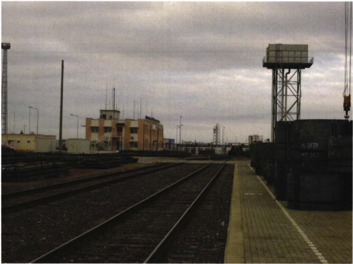
Rear railway and AISC office
