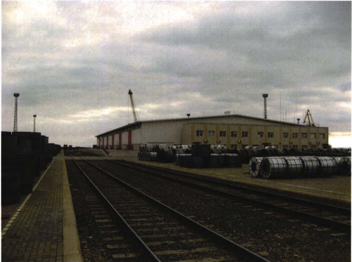
Railway behind shed
