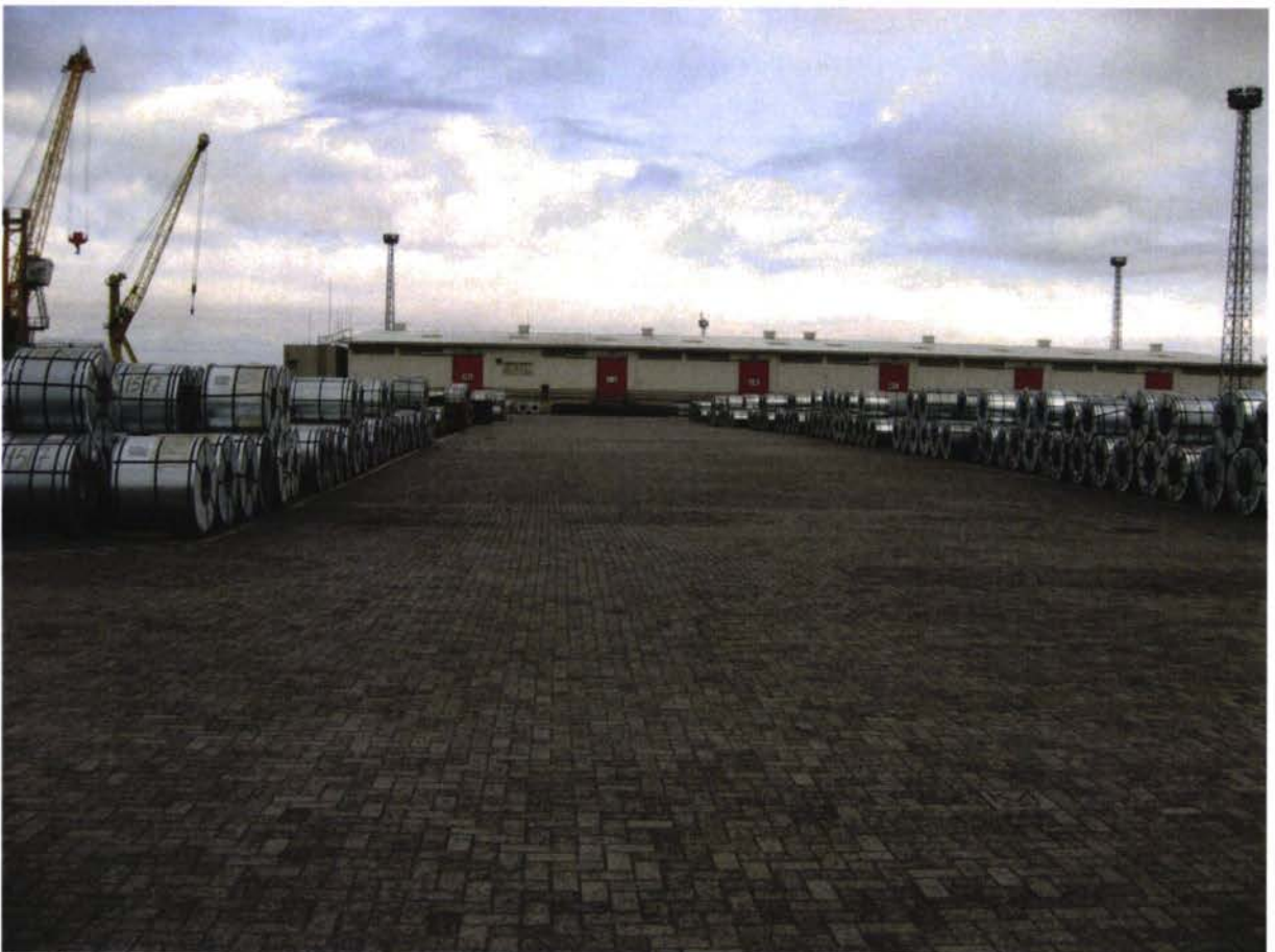
Steel stackyard behind berths 1-3 (shed at rear)
