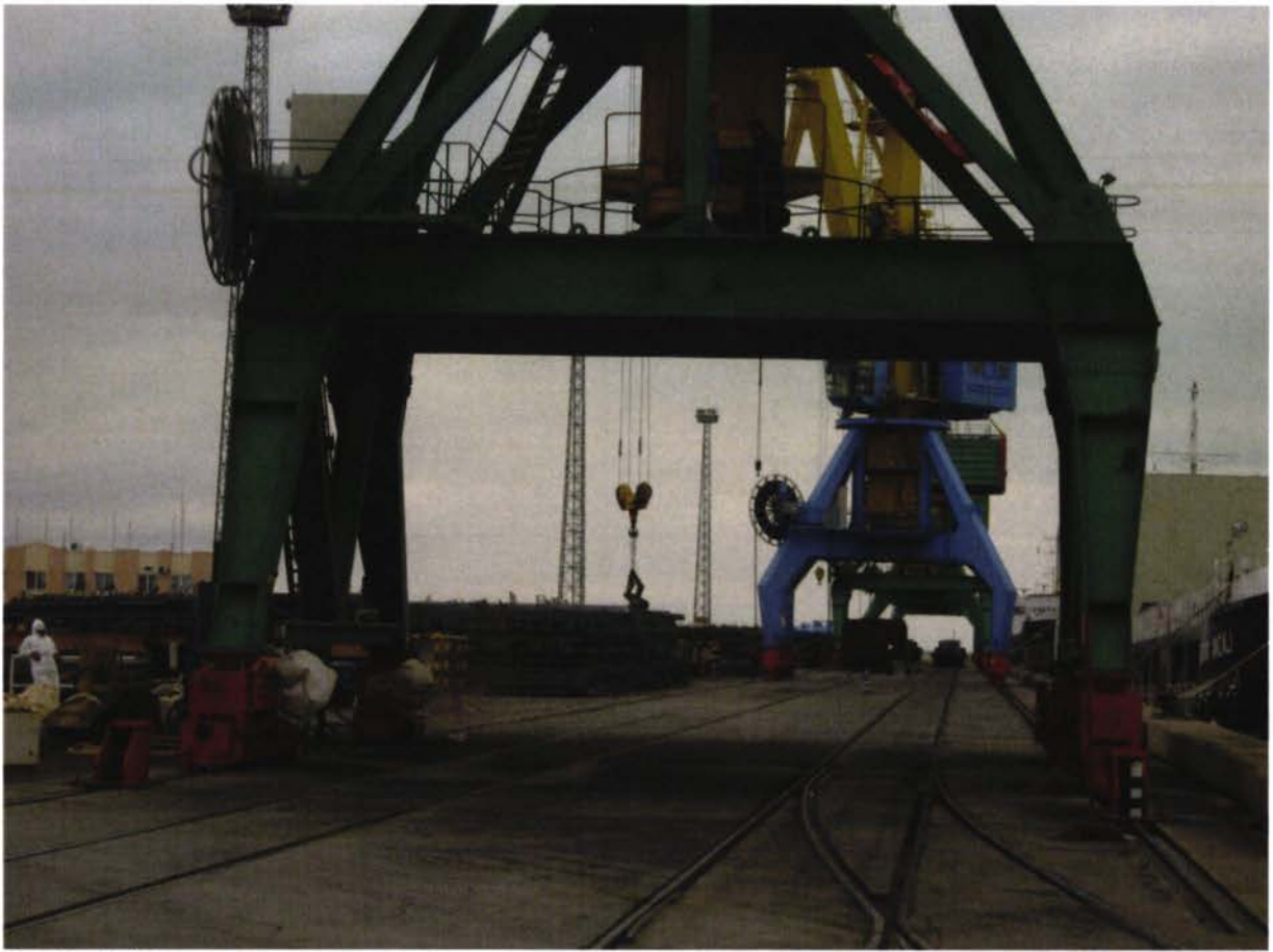
Berths 1-3 quay apron
