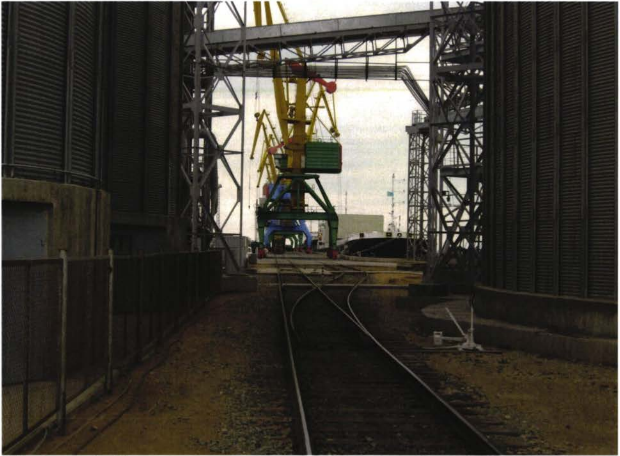
Railway at grain silos
