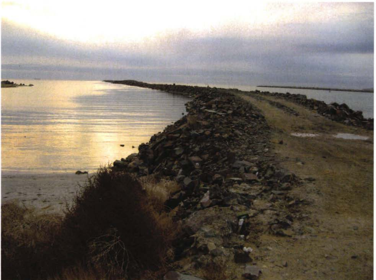
North port breakwater
