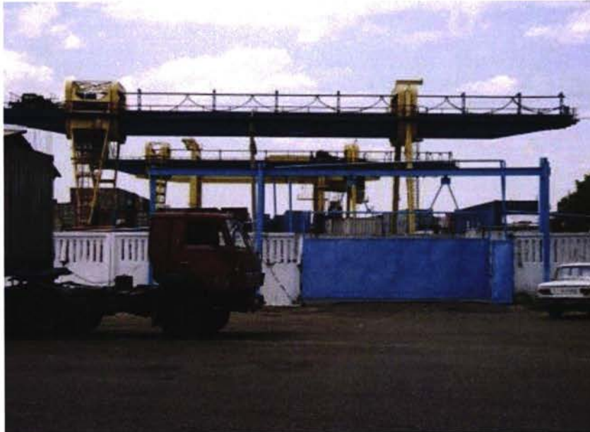
Photo 5.4. Railway Terminal Chukursay
