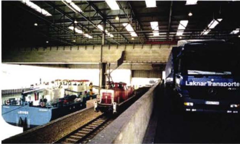
Figure 11.8 Trimodal Transshipment Terminal, Port of Duisburg: Haeger & Schmidt
