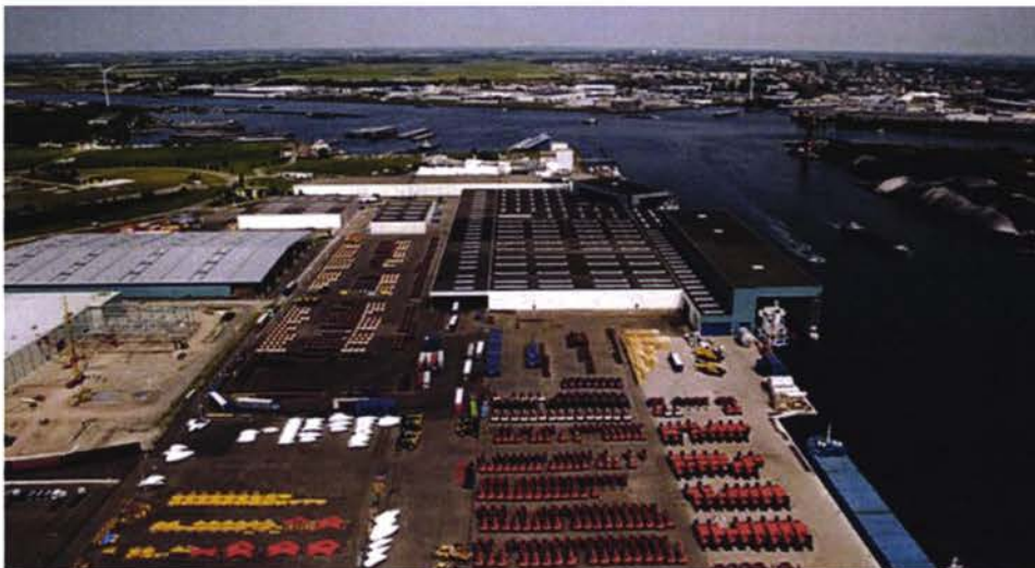
Figure 11.9 Overview Waterland Terminal, Amsterdam, NL
