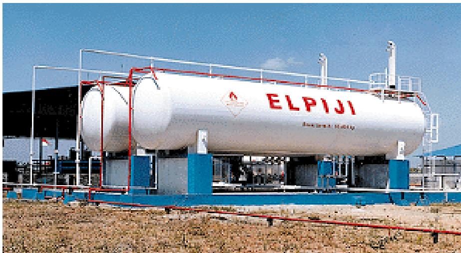
Figure 2.2 LPG storage tanks of approximately 1,000 mT - common type in the CIS ('cigar')
