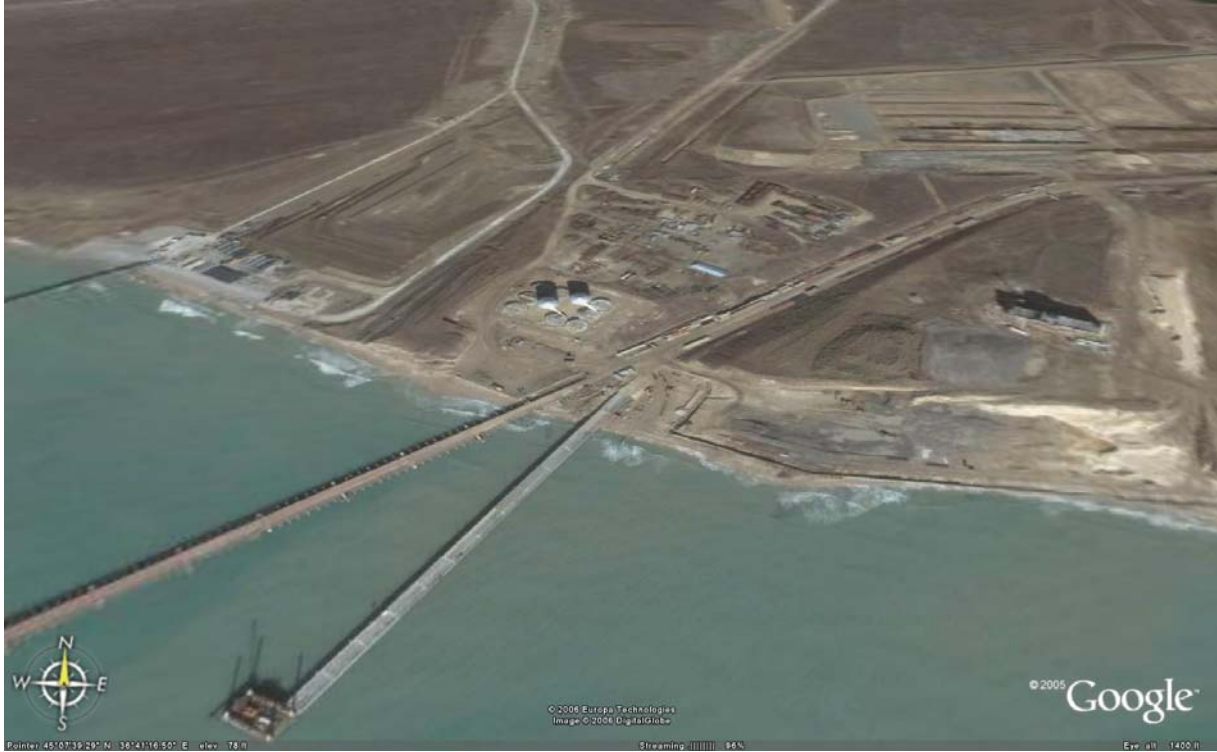
Figure 3.7 Taman port under construction
