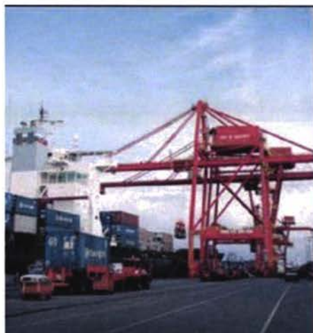
Ship-to-shore gantry cranes
