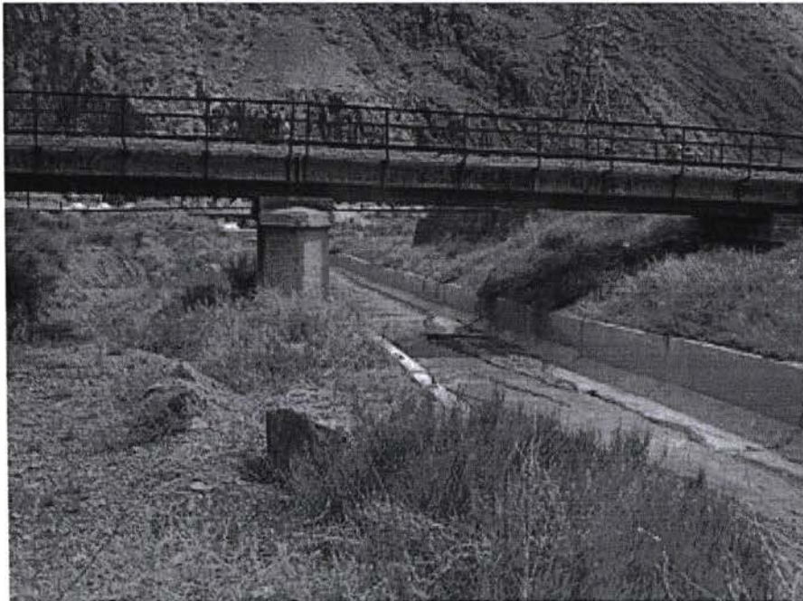
Fig. 2.5 – 2 - Old concrete channel along the river bed
