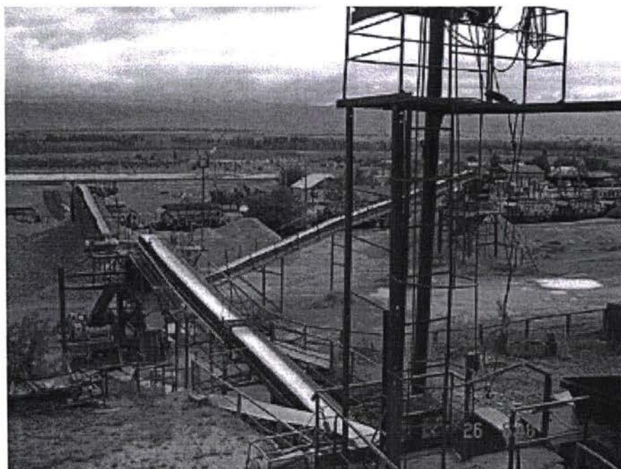
Figure 2.7 - 2 – Existing crushing plant
