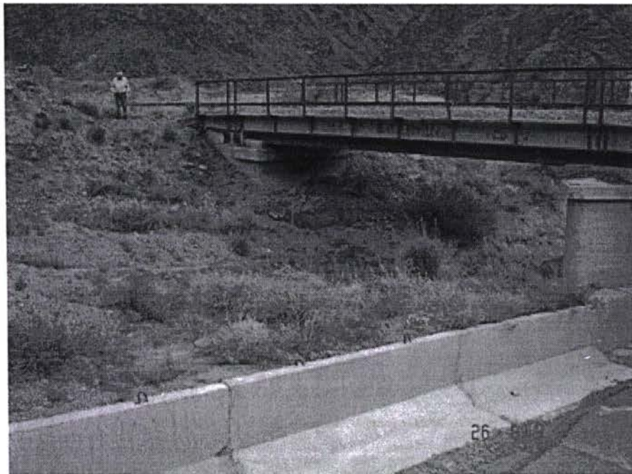
Fig. 2.5 – 1 – Bridge after Djil Aryk
