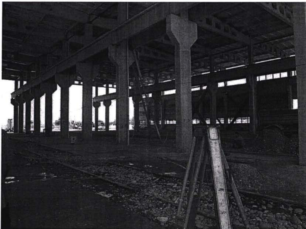
Photograph 6 – Kurgan-Tyube depot – Main maintenance building
