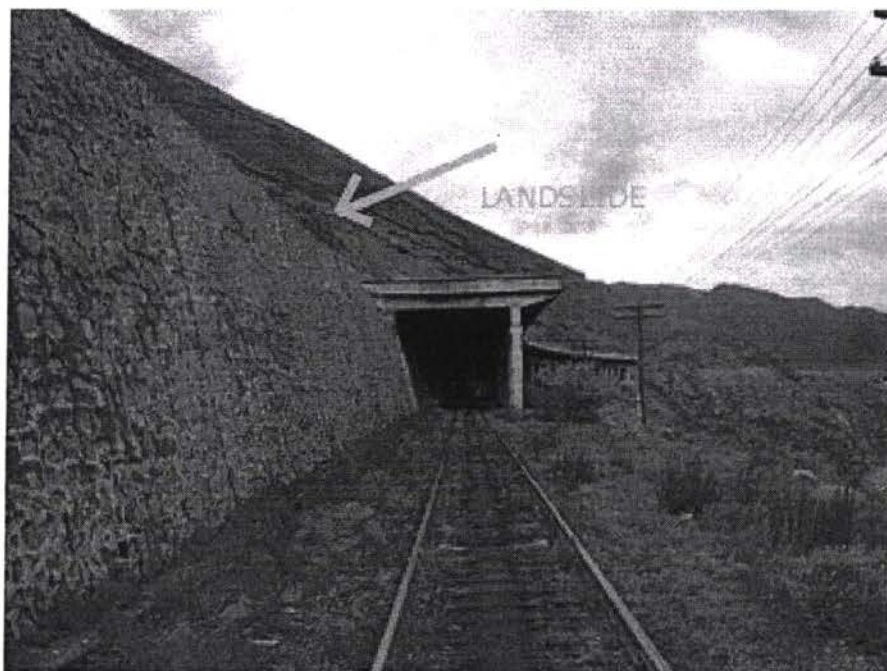
Figure 2.6 - 1 – Avalanche shed with landslide on the back
