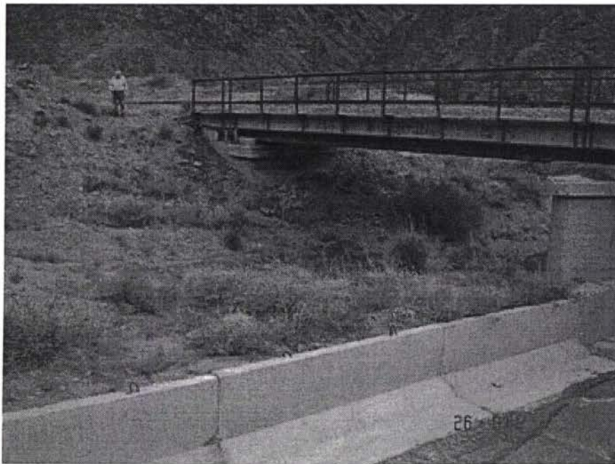
Fig. 2.5 – 1 – Bridge after Djil Aryk
