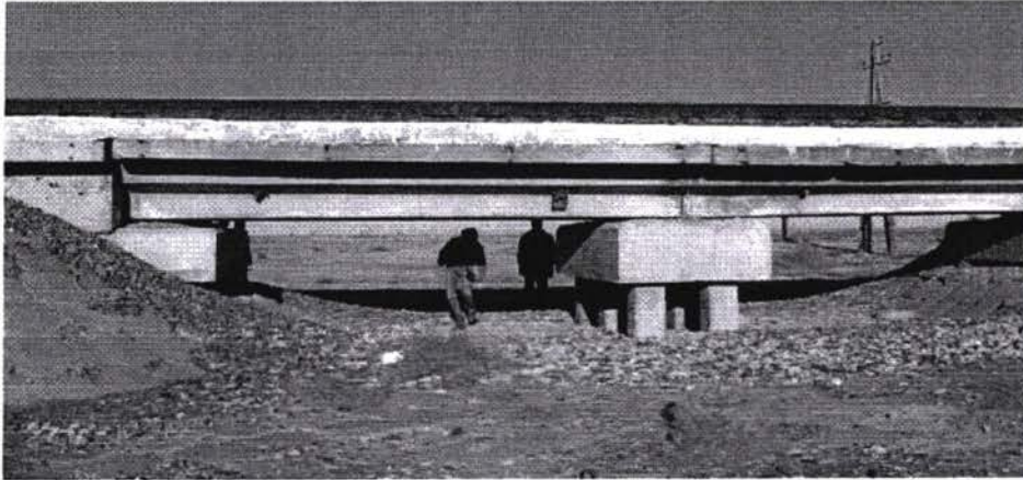
FIG. 26 Structures. 2 by 6m span hydraulic bridge.
