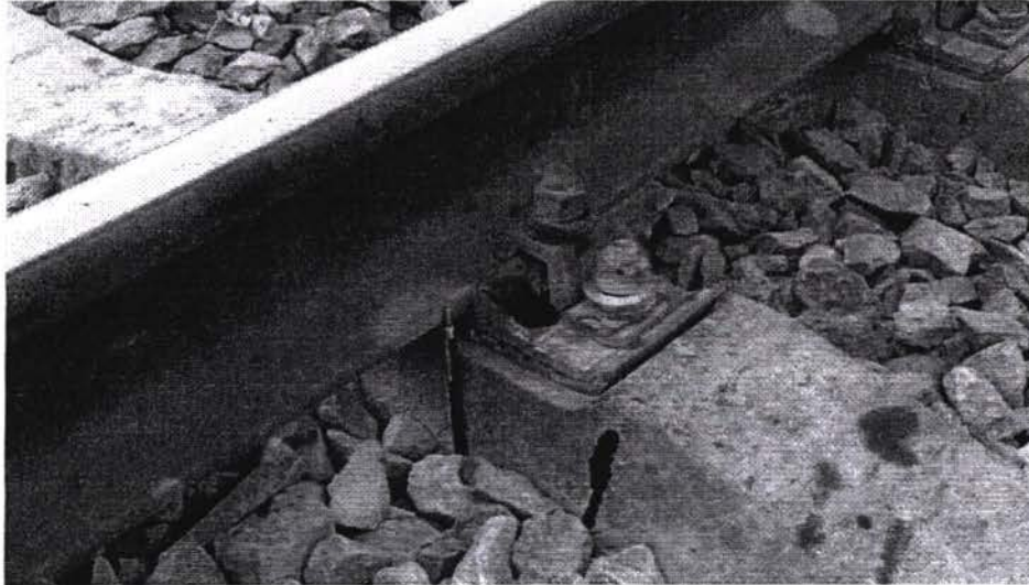
FIG. 1 Permanent Way detail: indirect standard fastening device.
