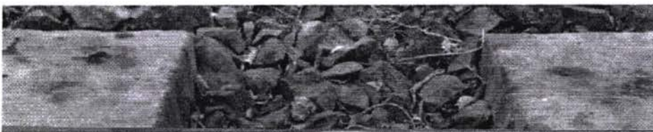
FIG. 5 Permanent Way detail in a renewed section (R65 and concrete sleeper): rail joint particular. The photo shows the excessive opening (3/4 cm). This phenomenon leads to the deformation of the rails heads for hammering effect of the train passage.
