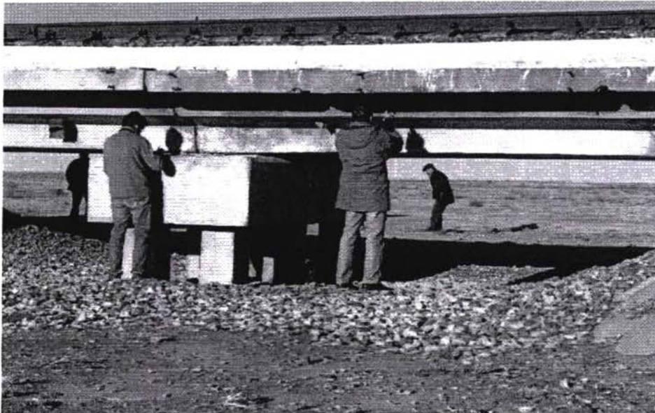
FIG. 29 Structures. 2 by 6m span hydraulic bridge.
