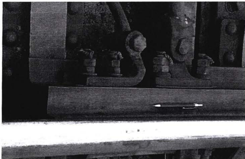
FIG. 13 Permanent Way detail: turnout. Particular of the closed blade.
