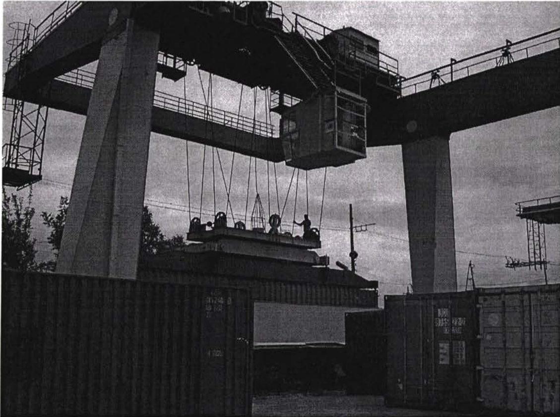
Figure 5 – Dushanbe terminal – Gantry crane lifting a 40' container
