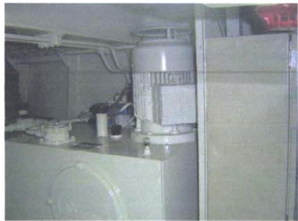
Hydraulic steering gear, tank and E-Motor for pump
