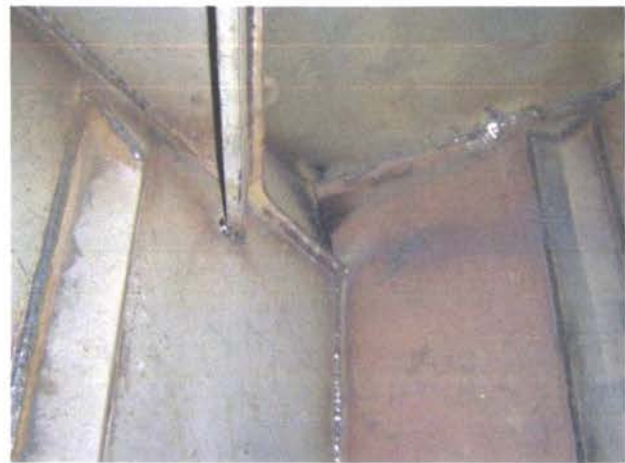
Welding on ceiling superstructure forward Port Side
