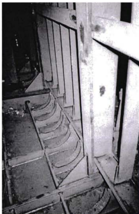
Frame setting of bow section, foreship still upside down
