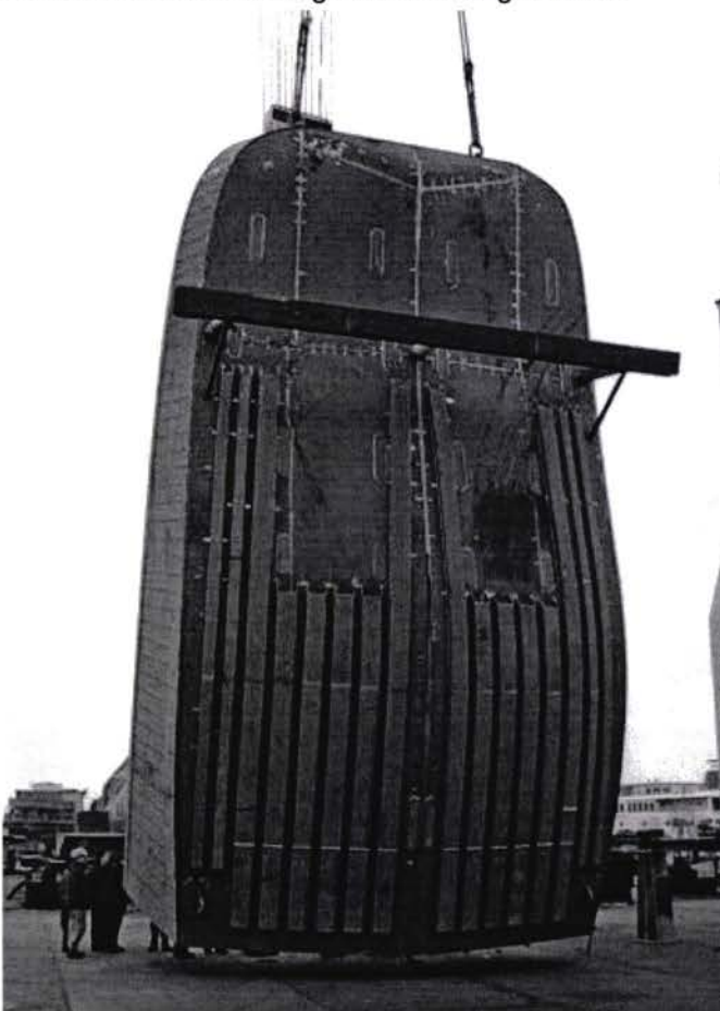
Bottom of aft section during turning
