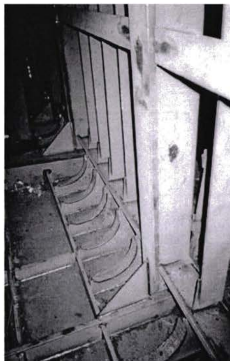
Starboard side shell frames with deck reinforcement brackets
