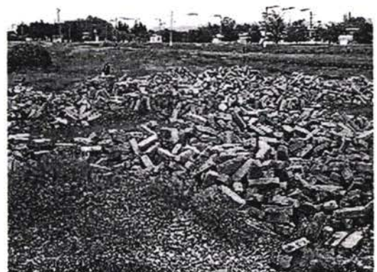
Kerbstones taken out under the existing asphalt layer between km 12+000 to km 20+680 and on stock pile
