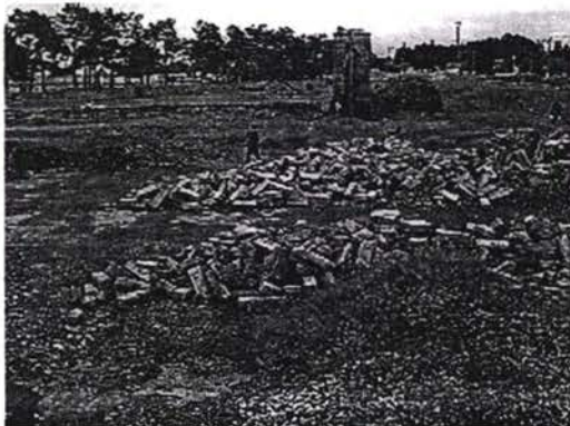
Kerbstones taken out under the existing asphalt layer between km 12+000 to km 20+680 and on stock pile
