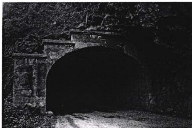
Portal from the tunnel exit
