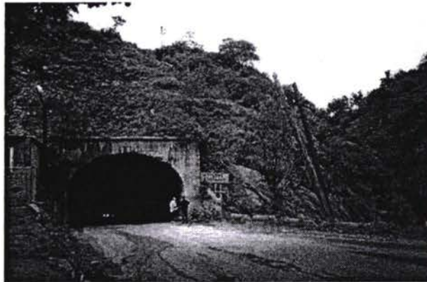
Portal to the tunnel entrance
