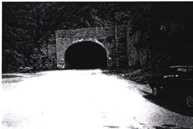
Portal from the tunnel exit.
