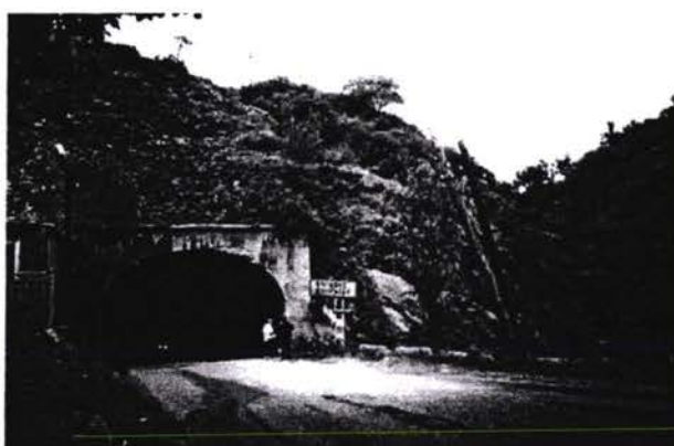
Portal to the tunnel entrance
