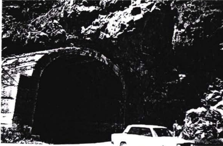
Exit from the tunnel
