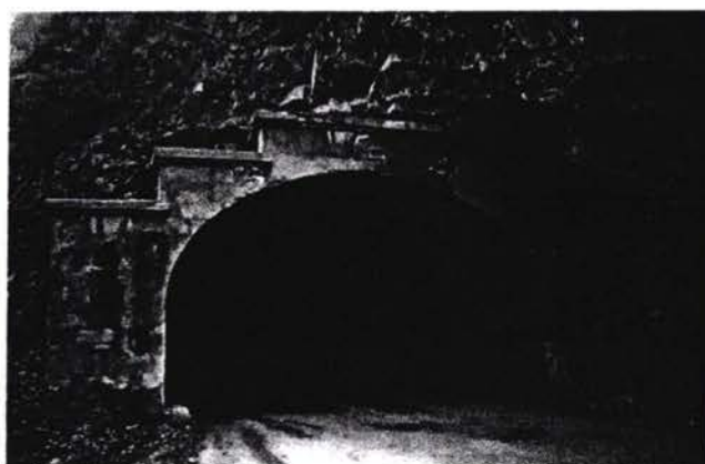
Portal from the tunnel exit
