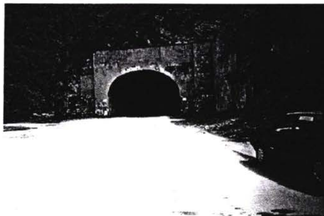
Portal from the tunnel exit.
