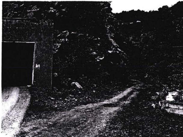
Tunnel 1. View of side road from South Portal
