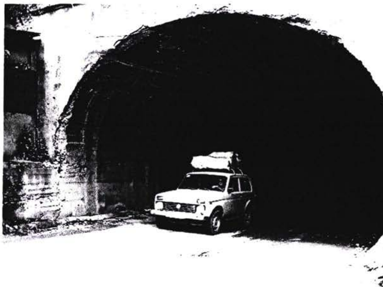
Tunnel 2. View of South Portal
