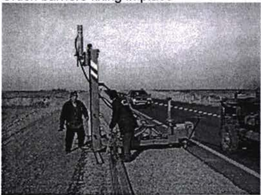
Crush barriers fixing in place
