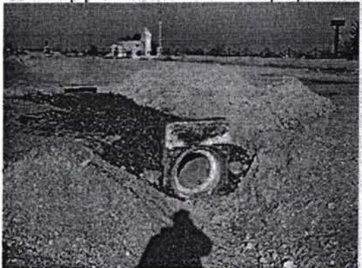
600mm pipe culvert – access to properties
