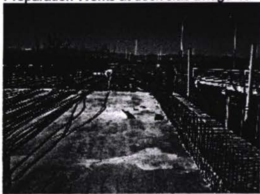
Preparation Works at deck slab Bridge 45
