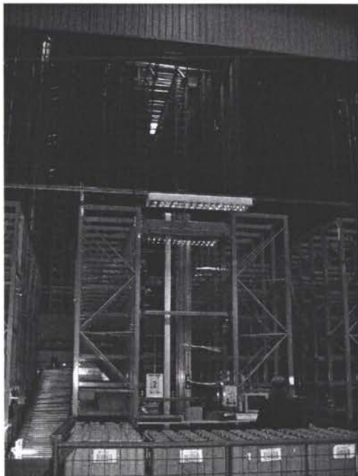
Automated handling – Autogerma
