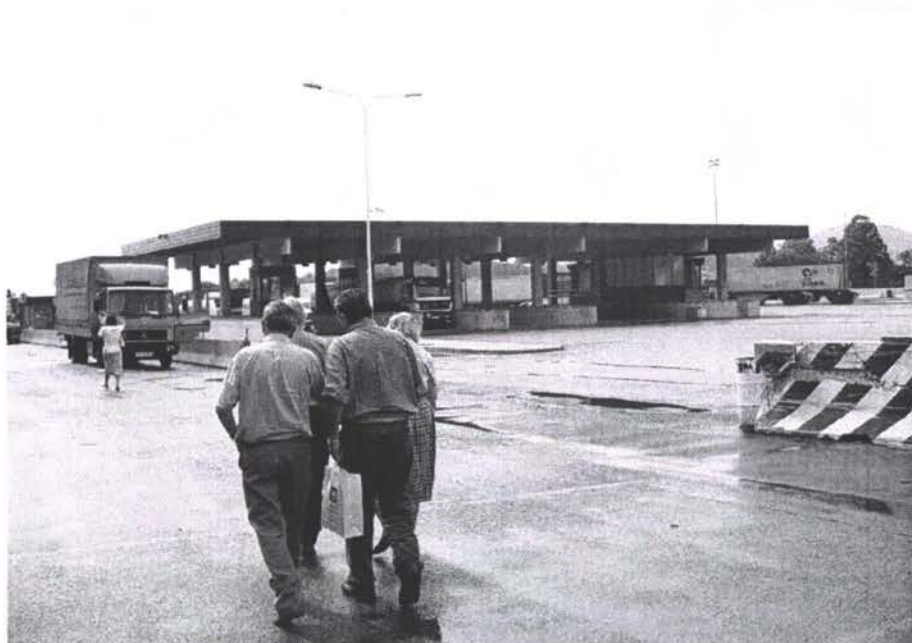
BTC freight terminal
