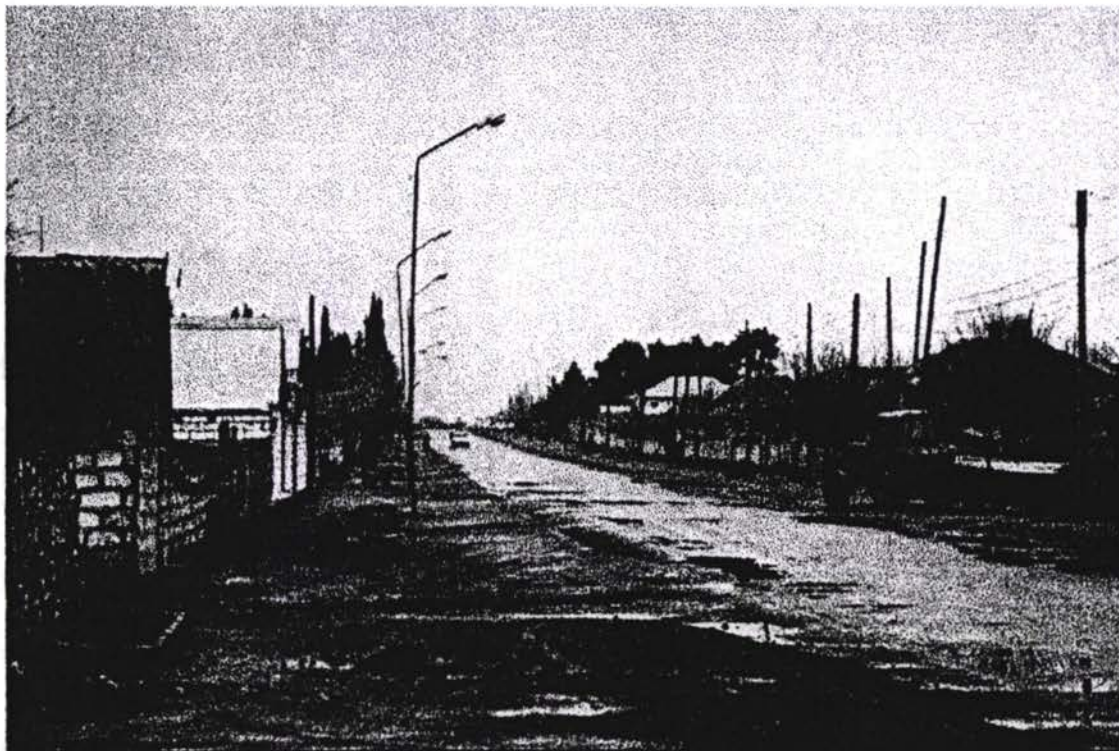
Photo 8. Settlement at about 20 kms distance from the border, sidewalks for pedestrians and drainage shall be prepared during the rehabilitation.
