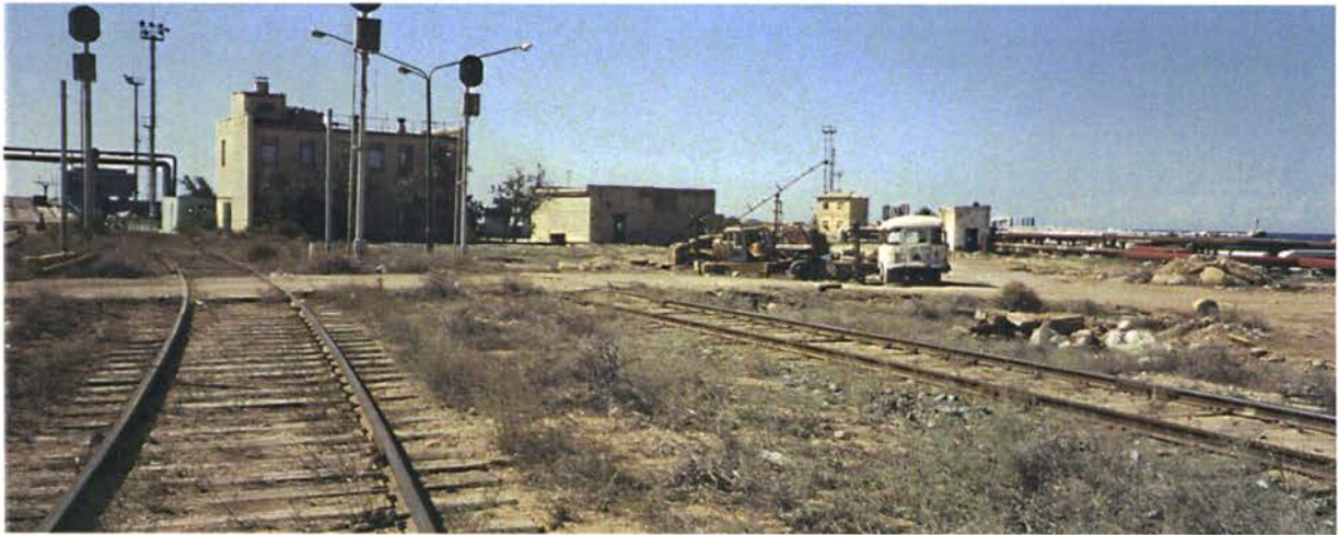
5- Morport railway station control building and transformer substation TP 803.
