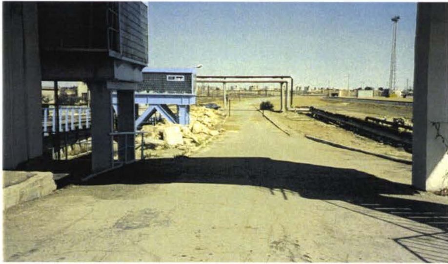
23- Access road to central pier.
