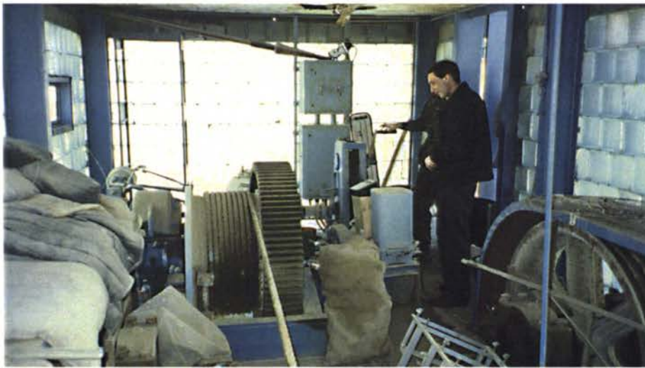
21- Inside an outer lifting tower.
