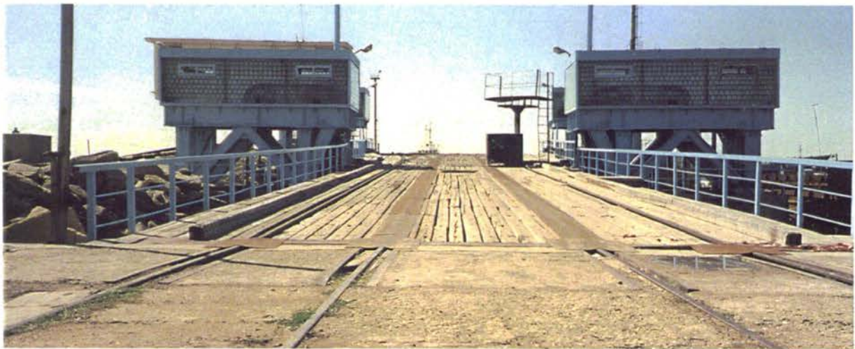
2- Two entrance rail-tracks, ramp deck and inner lifting towers.
