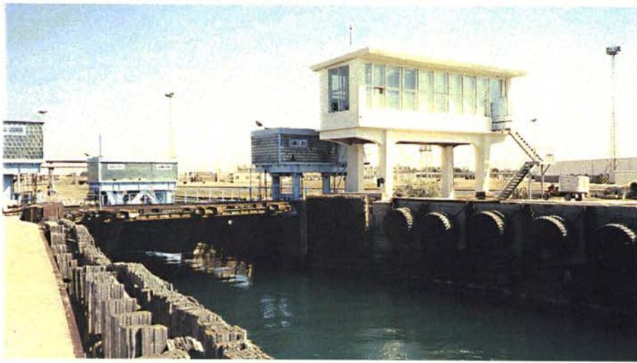
18- Central control tower and front end of the ramp.
