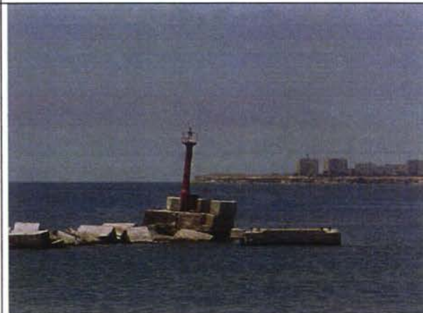
Starboard side port entrance, end of breakwater
