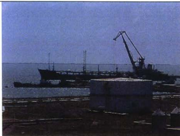
View from Administration Building to pier 3 and berth 4
