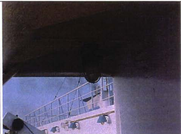
Ceiling lamp near lifeboat station, out of order
