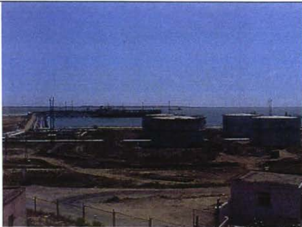
View from Administration Building to pier 1,2,5 and tanks pier 1,2,5 and tanks
