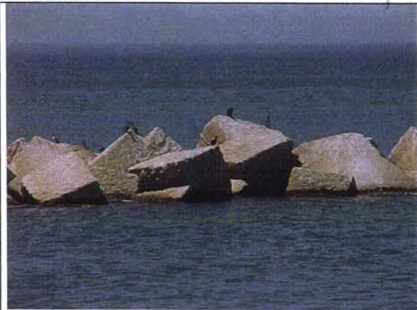
Breakwater , west side
