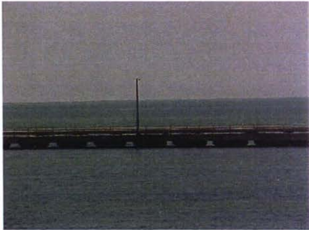
Pipeline to oil terminal with out breakwater in the south
