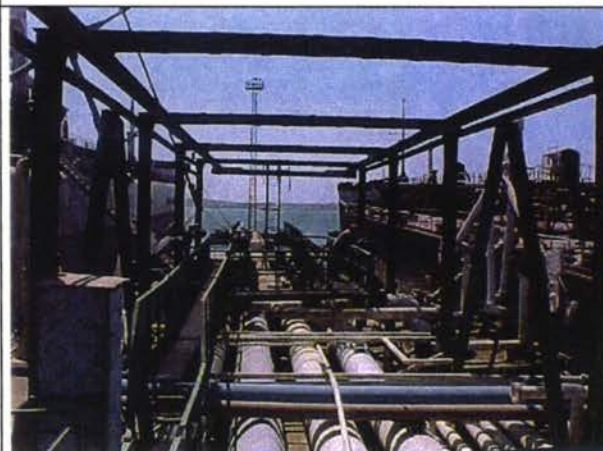
View to pipeline system on pier 1
