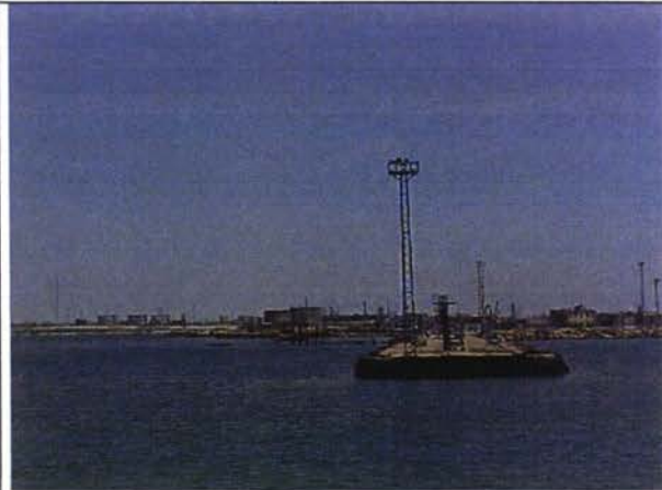
Port side port entrance, old oil terminal
