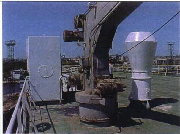
Both life raft cranes are without electrical support, cables are broken, not useable
