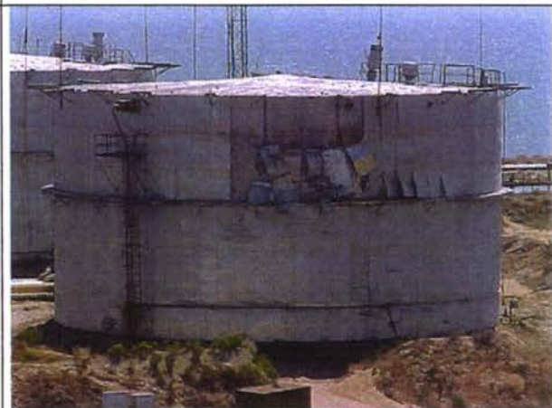
View from Administration Building to oil tank, low maintenance
