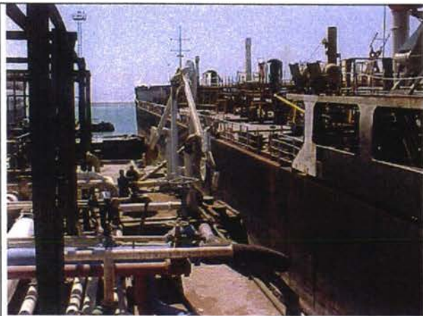
View to tanker " General Heydarov", 4987 t, with disconnected arms
