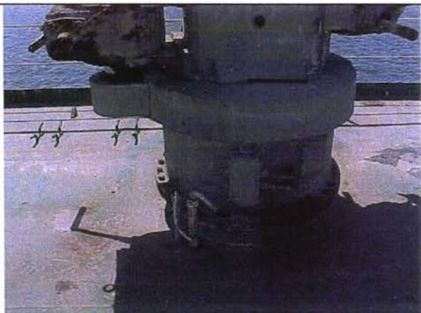
Both life raft cranes are without electrical support, cables are broken, not useable
