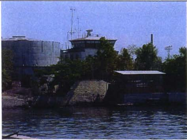
View from berth No. 9 to harbour and coast control. Water tank for fire fighting system
