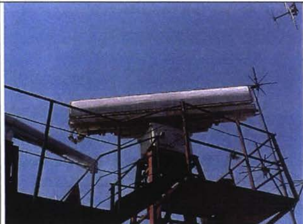
Antenna for three and 10 cm Radar from Radar control centre of harbour and coast area
