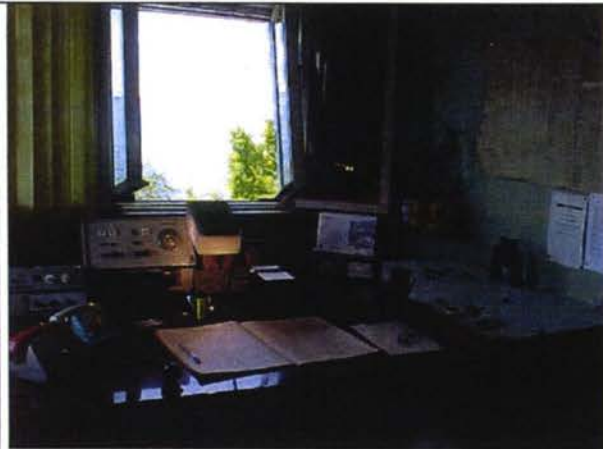
Radio room from Radar control centre of harbour and coast area, only VHF, no GMDSS
