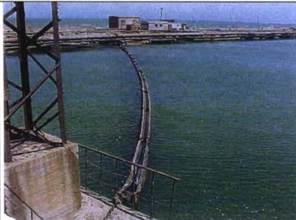
Oil boom, in stand-by position, not around discharging tankers
