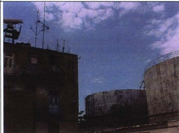
View to Radar control centre of harbour and coast area with water tanks for fire fighting system and port supply.
