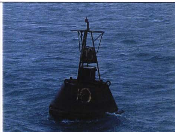
Port buoy 10, without topmark and red colour nearly off, damaged fender
