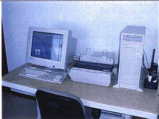
Computer for Buoys and Leading Lights control system
