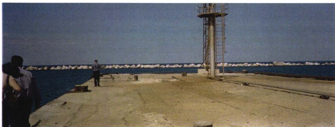
8. Head of pier: second water cannon and floodlighting lattice tower in the back (June 2001)
