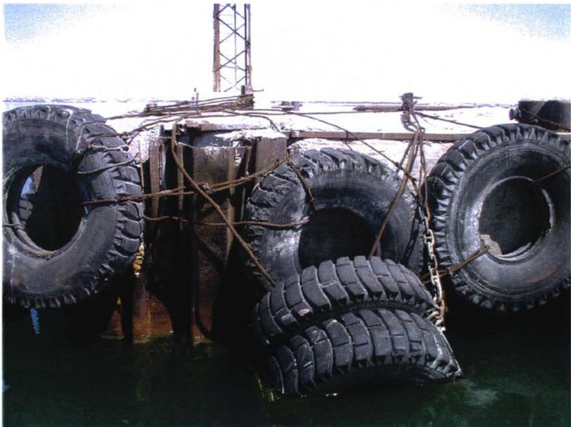
2. Fenders hanging from pier head, inner side (June 2001)
