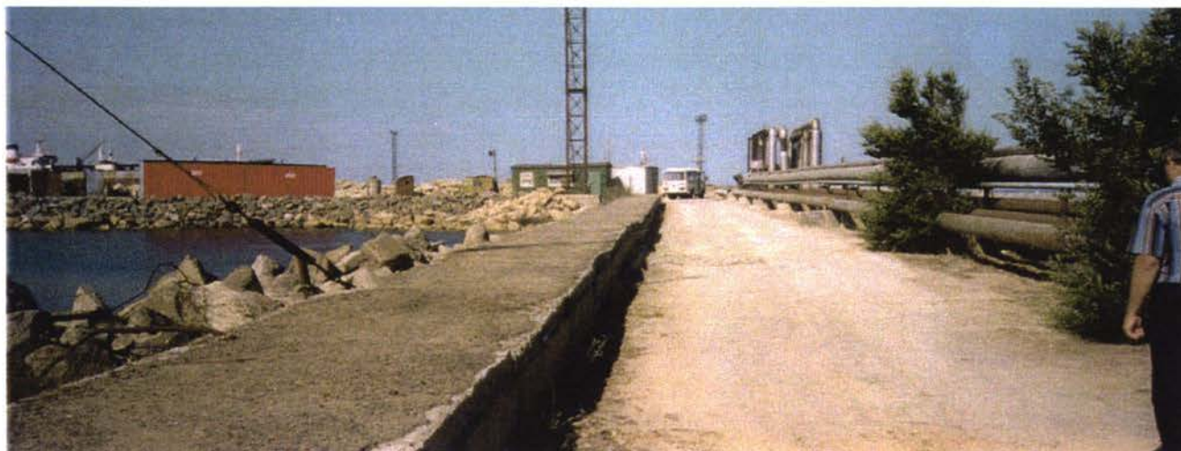
9. Access causeway, towards the pier (June 2001)
