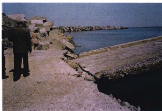
3. On the breakwater. Connection with pier n°5
