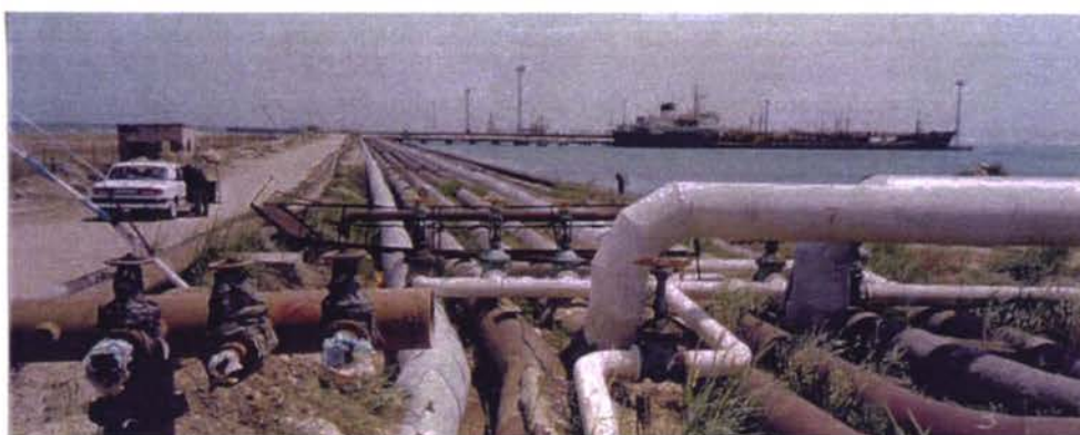
2. The breakwater, from its root, and pier n°1
