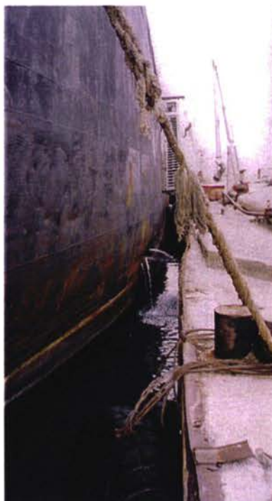
3. Berth n°5. Details of capping beam, bollards, mooring ropes and fenders
