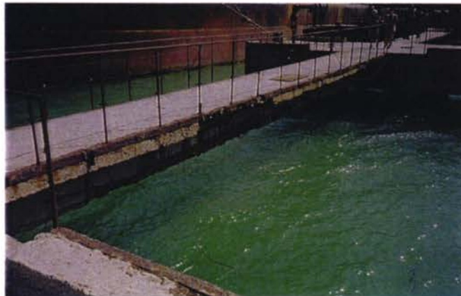
11. A pedestrian bridge on pier n°1
