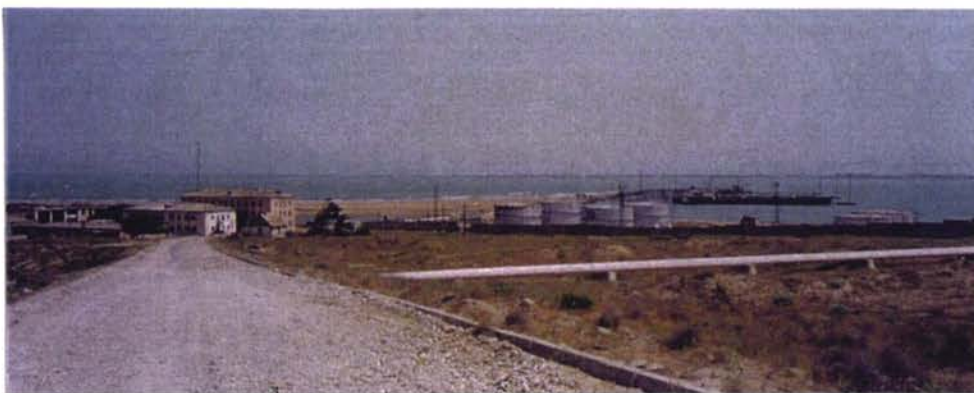
1. General view of Dubendi Oil Terminal, seen from the upper tank-farm area
