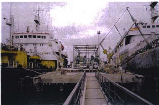
8. On pier n°1
