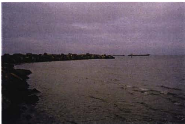
7. Head section of the breakwater (notice sheet piles)
