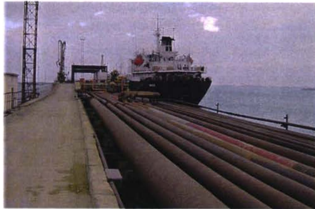
14. Access causeway to pier n°3
