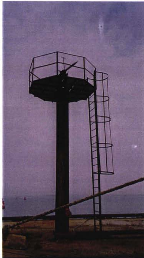
5. Fire-fighting tower between berths n°4 and n°5
