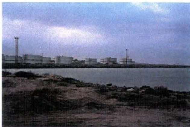
23. Lower tank-farm (northern part)
