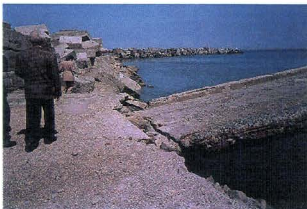
3. On the breakwater. Connection with pier n°5
