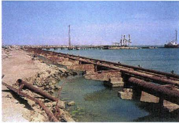
4. Along the inner part of the breakwater (oil pipe supports)
