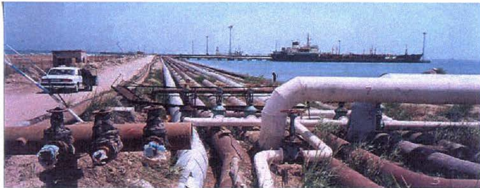
2. The breakwater, from its root, and pier n°1
