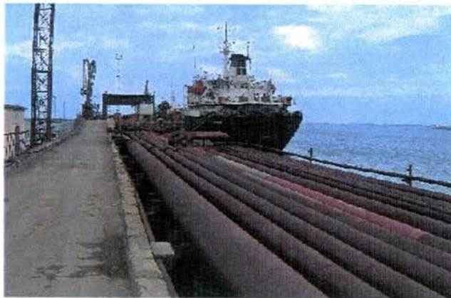
14. Access causeway to pier n°3
