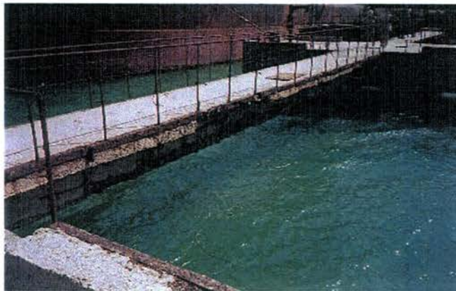
11. A pedestrian bridge on pier n°1
