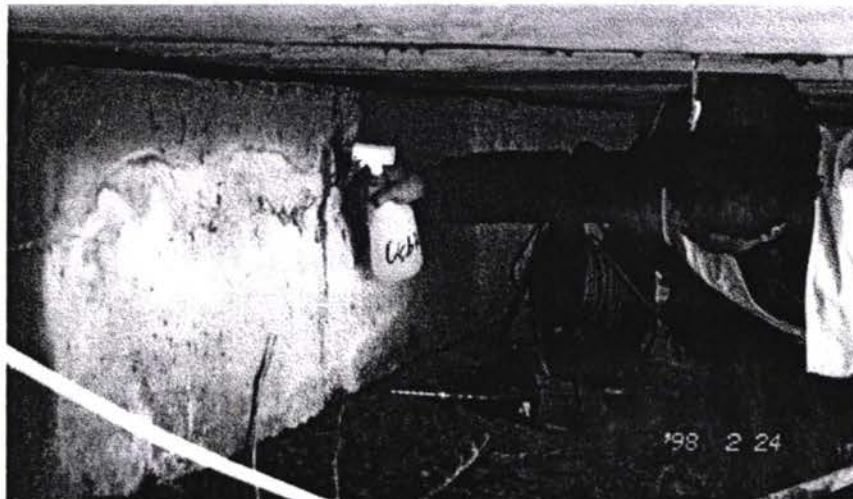
Testing for chloride penetration using Phenolphthalein indicator, Tashkent, Uzbekistan.
