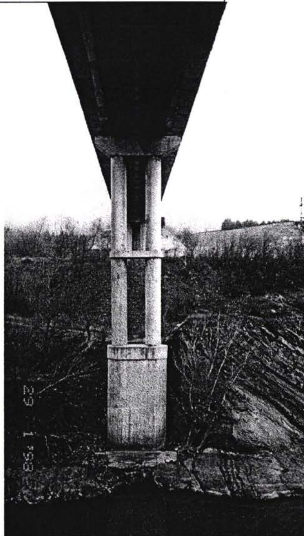
Steel plate girder viaduct examined, Georgia. Ref S-12 Br 2 km 3+905
