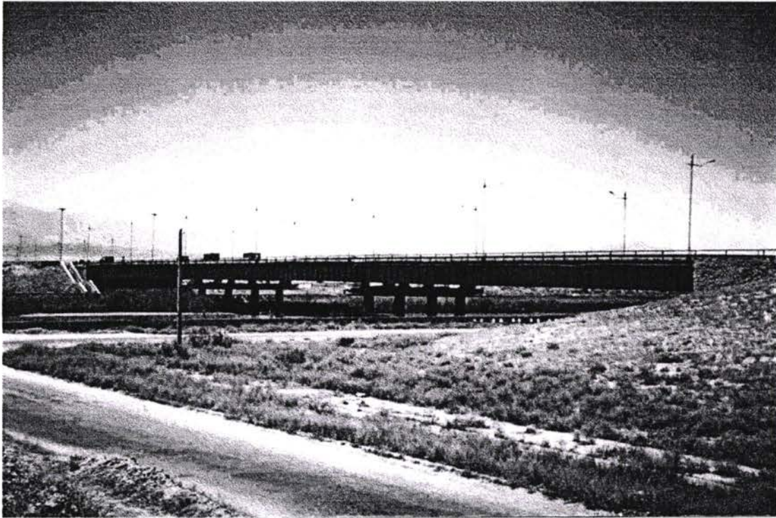
3 Bridge over the Kara-Kum Canal, assessed for strength
