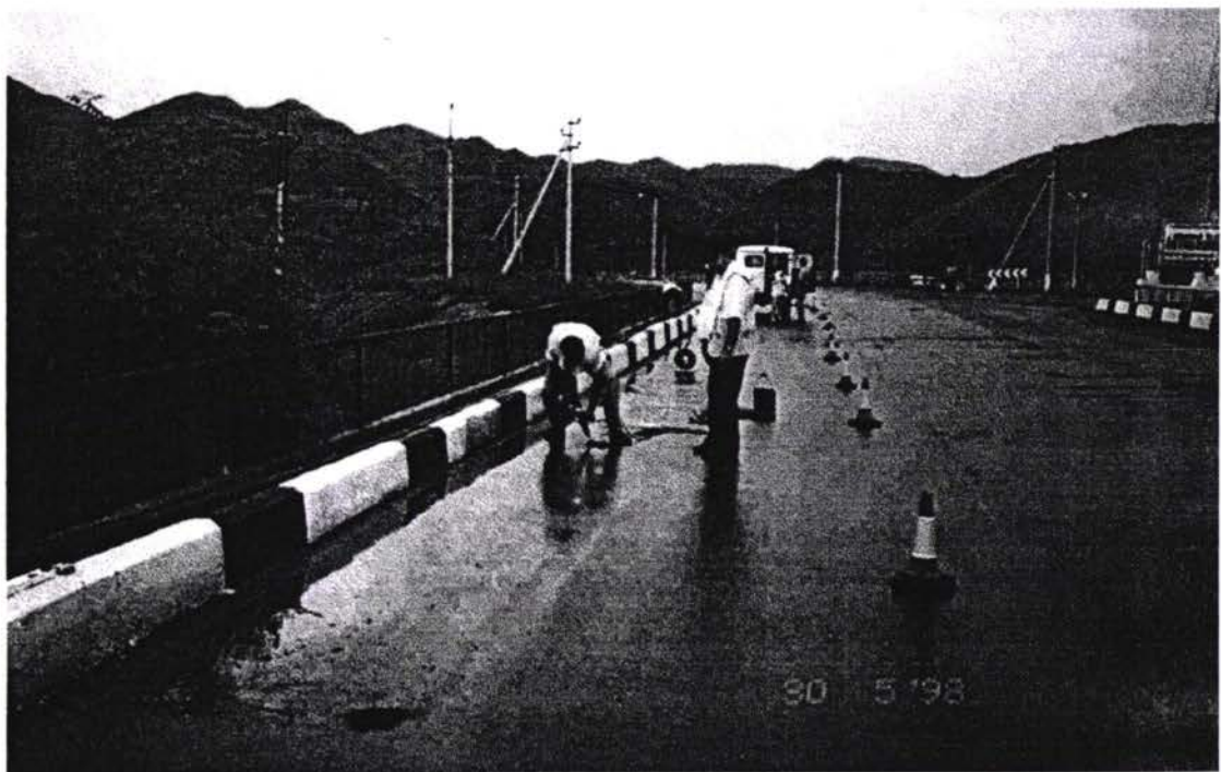
6 Establishment of surfacing thickness for bridge assessment purposes, Turkmenistan
