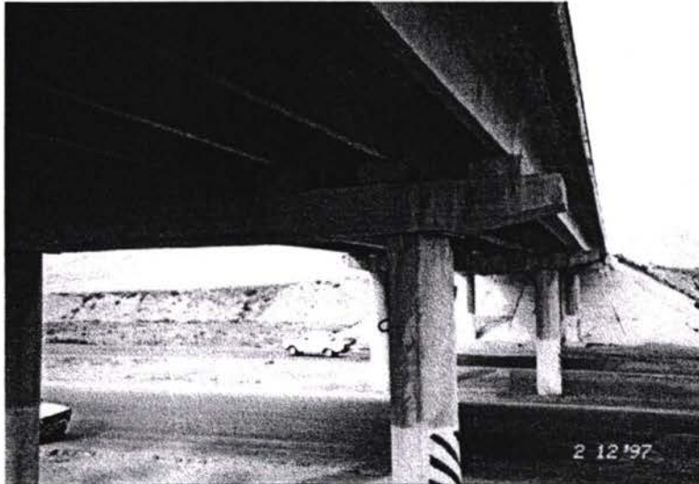
Typical structure examined, Baku , Azerbaijan. Bridge 3 Astara-Baku km 267+342 Karadagski region
