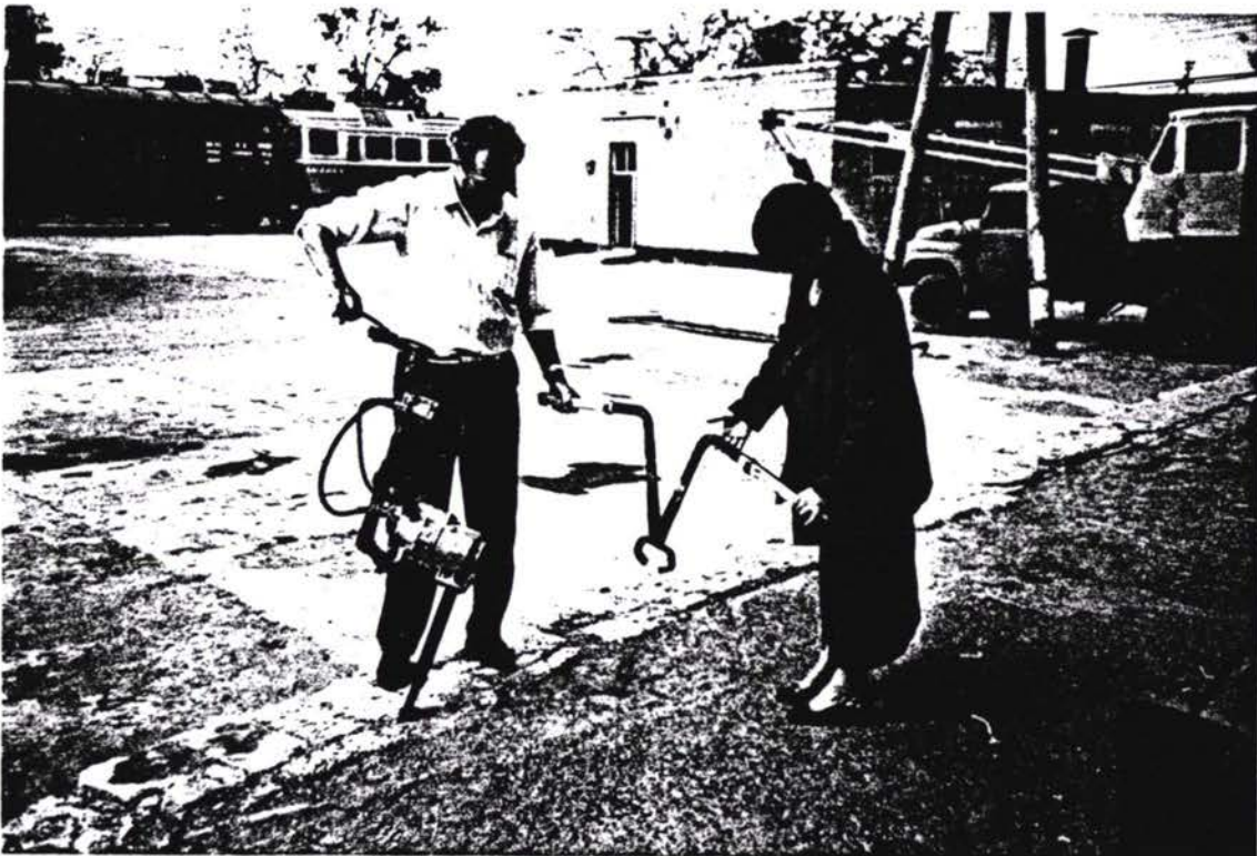
Existing tamping machine and rail lifter
