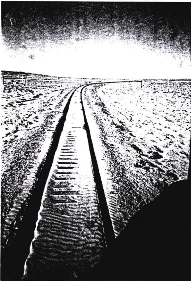
km 328 A linepart with sand in the track
