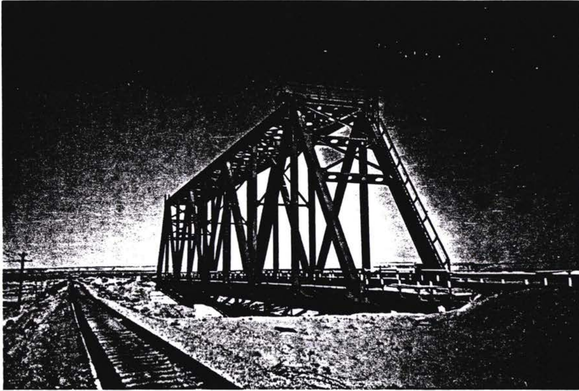
Bridge at km 39,9 Eosion at the river bed
