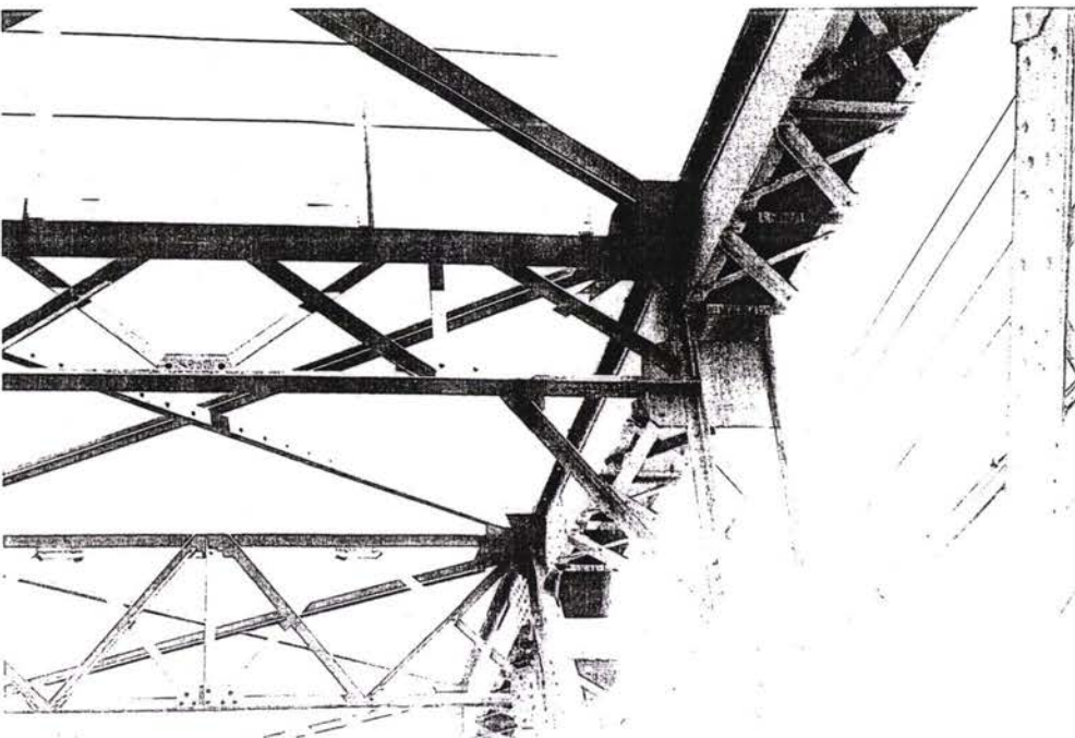
F6-18 Span 13 Bracing angle out of axis
