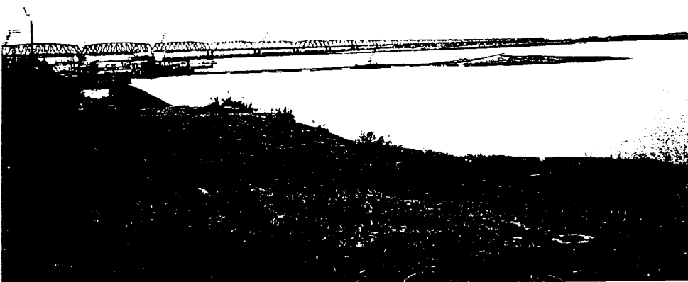
F5-30 View of the existing bridge
