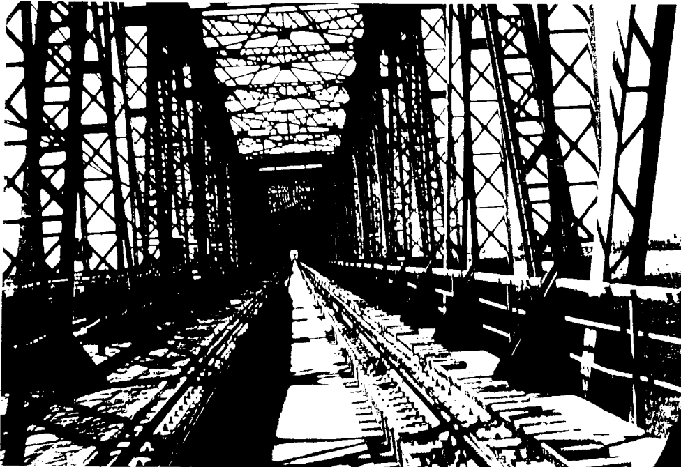
F6-26 Span 13 View along bridge inside
