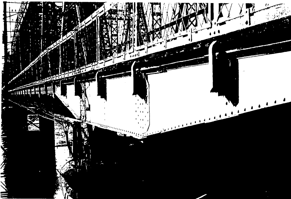
F7-25 Span 26 Footbridge US
