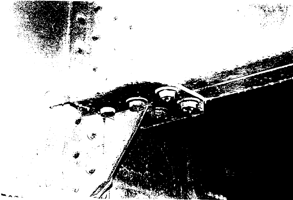
F7-33 Span 25 Reinforcement of crossgirder
