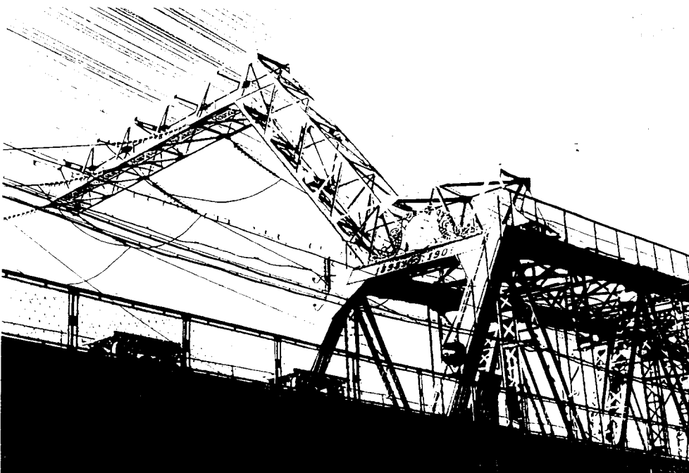
F9-07 Span 1 End frame with high voltage line
