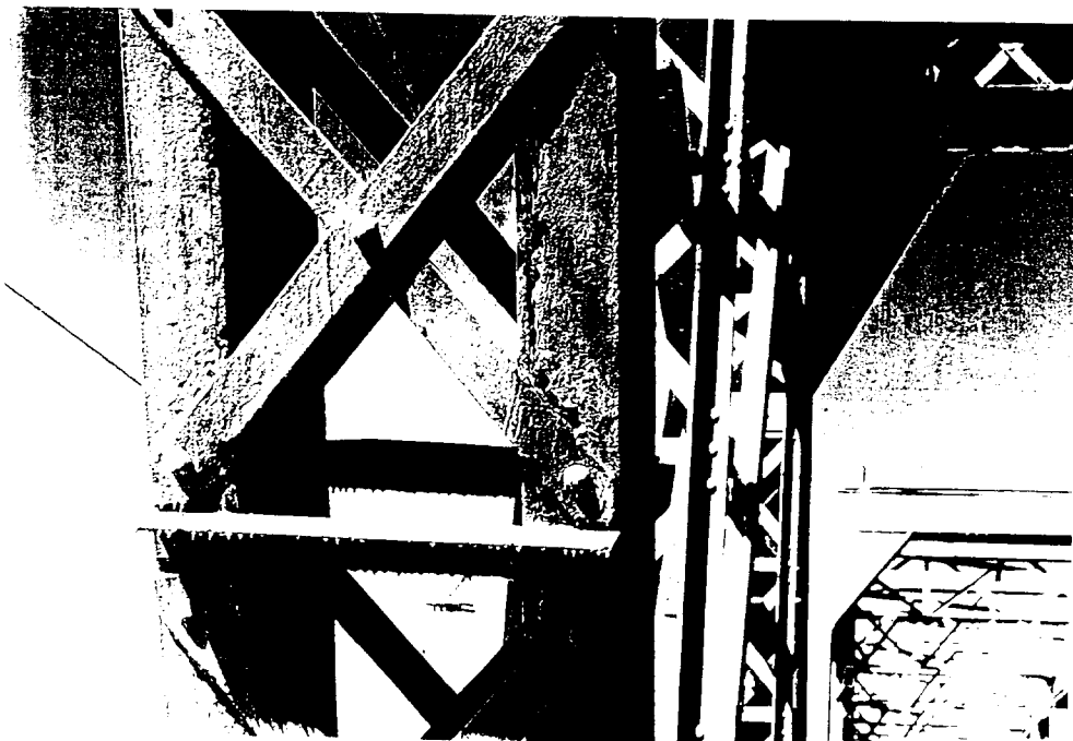
F6-37 Span 13 Corrosion of dia- gonal
