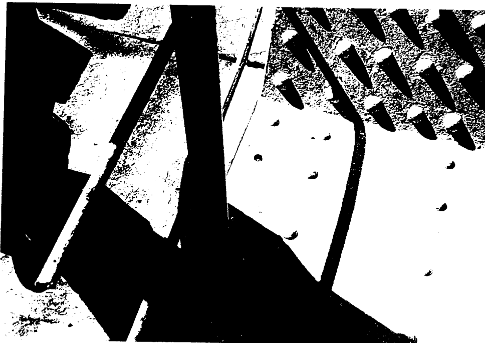
F4-21 Span 23 Missing rivet at end girder
