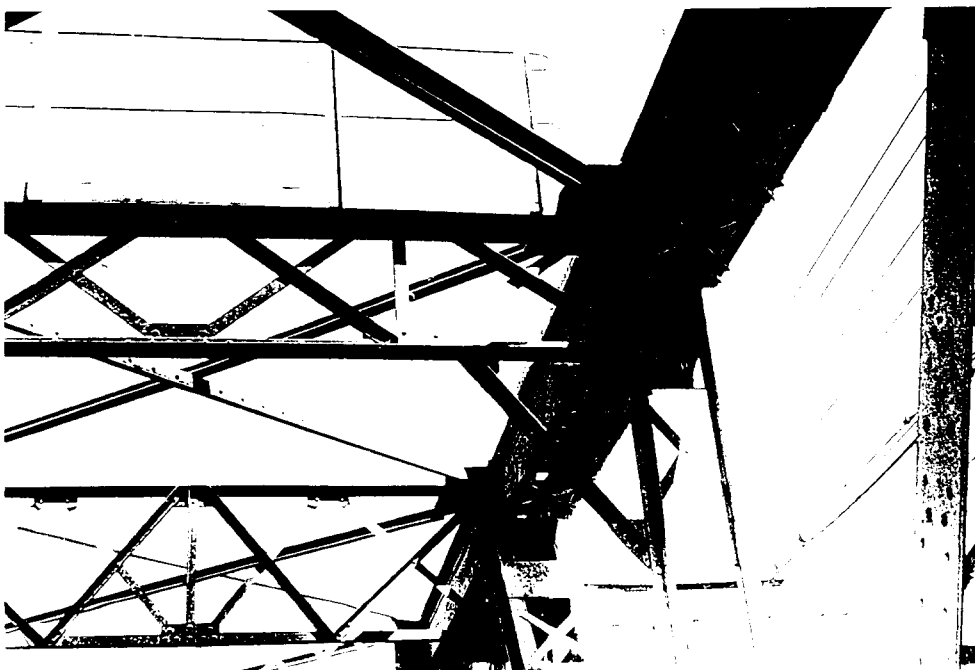
F6-18 Span 13 Bracing angle out of axis
