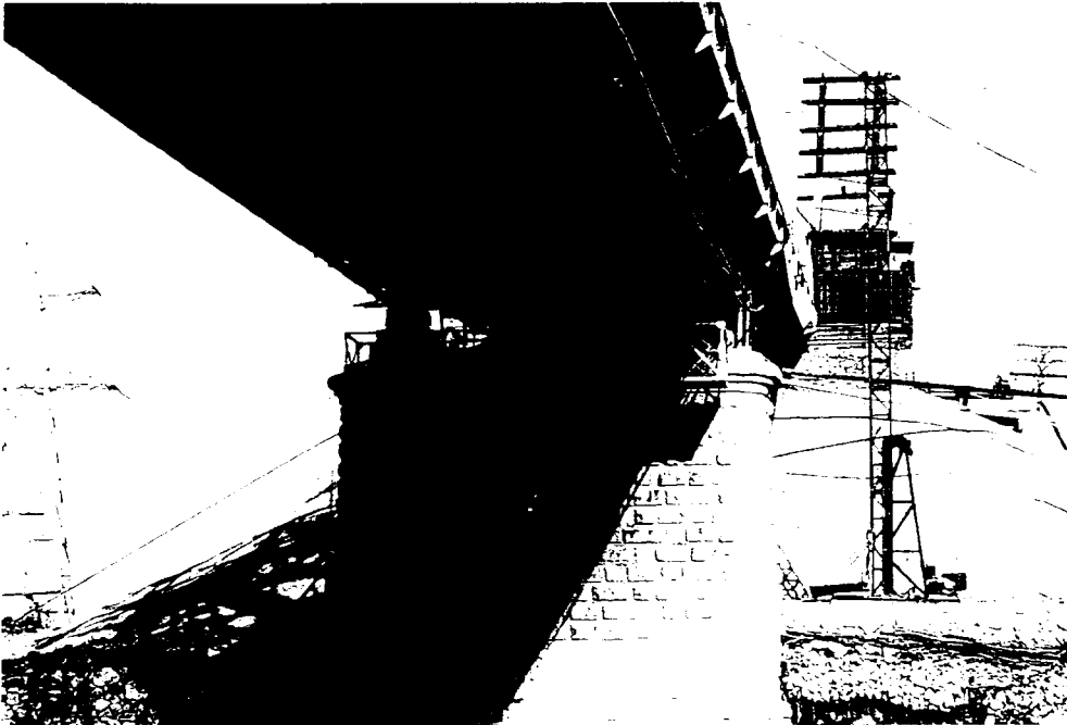
F8-21 Span 25 Bridge with guard room
