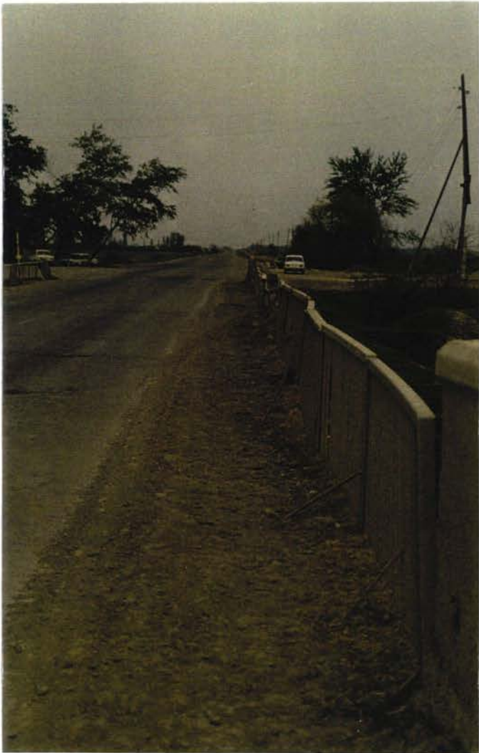
Fig. 8, 9 and 10: Safety deficits at the bridge near Sigirli: railings are dilapidated and too low, fixing inadequate and dangerous
