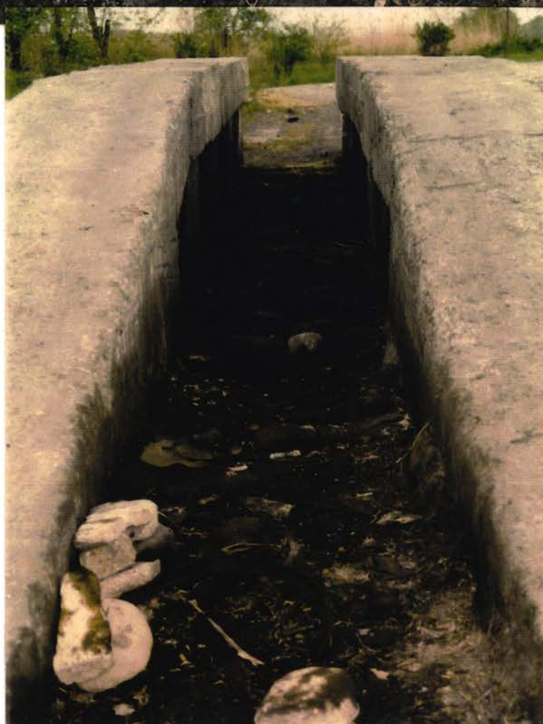
Fig. 5, 6 and 7: Vehicle repair ramps on the M 4: permanent sources of pollution with oil and waste and probably other harmful substances and waste
