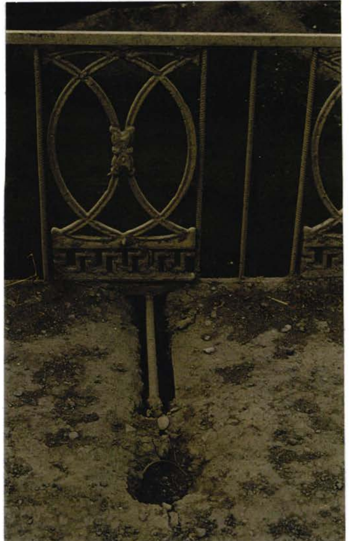
Fig. 8, 9 and 10: Safety deficits at the bridge near Sigirli: railings are dilapidated and too low, fixing inadequate and dangerous
