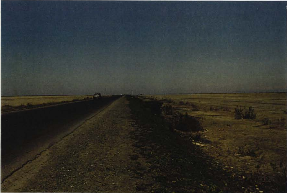
Fig. 1: Mugan desert: typical aspect of the road environment in the eastern part of the project area
