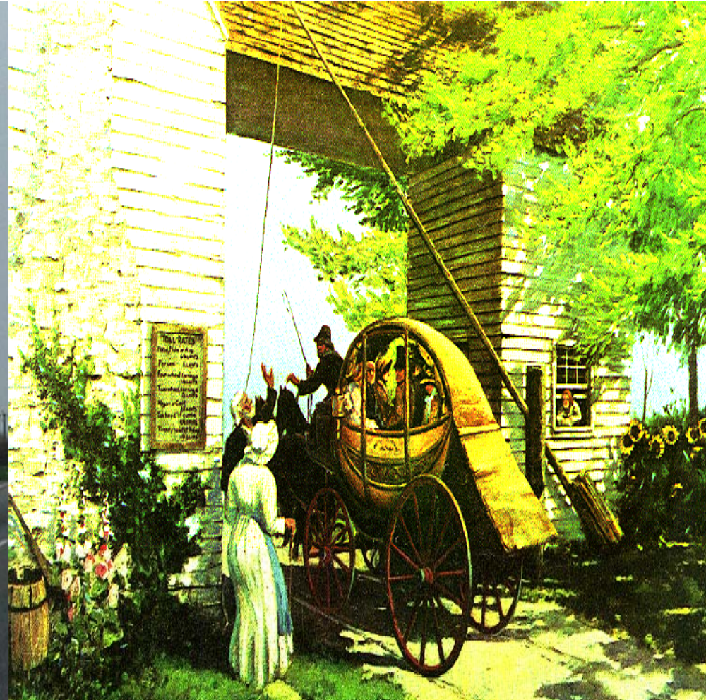
The Maysville Turnpike, USA, 1830
